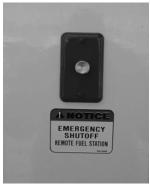
Turn ON switch on transfer pump and begin fueling
